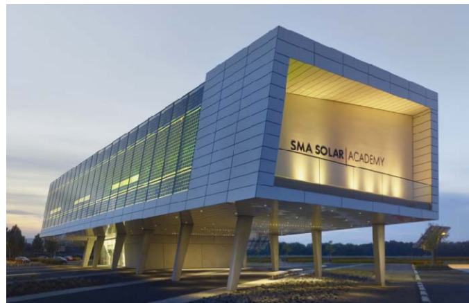
Figure 5: The “Solar Academy” in Niestetal (DE), design: HHS Planer + Architekten. The 1400 m 2 building was built in 2010. The idea of an “island operation” increased the PV capacity. The combination of façade, roof-top and on-site trackers ends in 152 kW p (complemented by a 70-kW el biogas CPH and a 230-kWh battery pack). Source: SMA, Constantin Meyer
