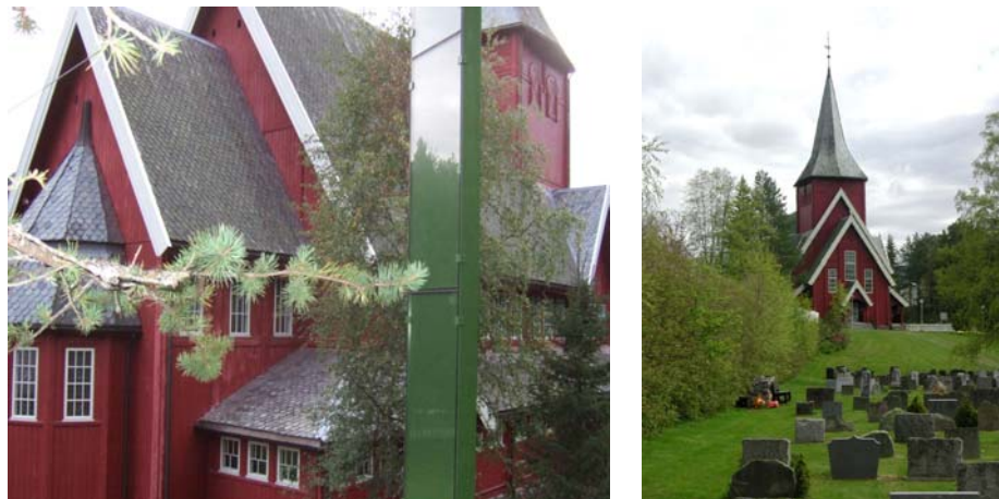
Figure 12: PV on building's site(listed building) / Hol Church, Geilo, NO, design: Harald Røstvik. What do you do when you for antiquarian reasons are not allowed to do anything on the built envelope? An extensive search for alternative solutions did lead to the circling in of using the extended space around the church for energy producing, solar absorbing, purposes. A vertical ST absorber at a distance to the building, as a sculptural feature. The solar absorbing sculpture was designed in dark green so as to blend with the green forest next to it and hence not steal too much attention from the red church it was supposed to serve. A dark green solar absorber is less efficient than a black one, but only slightly and the loss in efficiency can easily be compensated for through increasing the solar absorber area by 10-15 percent. Source: H. Røstvik
