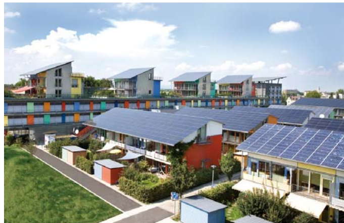
Figure 2: Net Zero Energy Buildings Cluster : Plus energy settlement in Freiburg (DE), design: Rolf Disch. The Plus Energy Settlement in Freiburg is an example where the zero energy balance is achieved in the frame of an estate. Some of the 59 built terrace houses have a positive, others a negative primary energy balance. The average is clearly positive. The efficient row houses are covered with 3150 m 2 of roof top integrated PV generators. The heat is supplied by district heating. The efficiency of the houses bases on the Passive House concept, and a consequent (urban) planning for shadow-free south orientation, position and shape of the buildings. Source: Rolf Disch.
