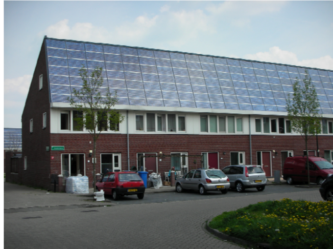
Figure 1: Nieuwland, Amersfoort (NL), 1999. Pitrus-Mattenbies project, design: Klaus en Kaan. 119 houses, showing 2462 m 2 PV used as roof cladding. Source: A. Scognamiglio
