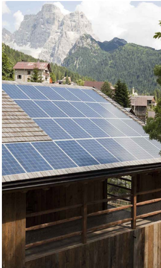
Figure 10: PV on building's (listed site) / Energy self-sufficient tabià (retrofit), Selva di Cadore (Belluno), IT, 2010, Design: EXiT. PV is part and parcel of the pre-existing wooden tilted roof. Tabià are named old buildings (XVII century) used as a stable or barn, which characterize the agricultural and pastoral architecture of the Selva di Cadore Valley in the landscape of the Italian Dolomites, classified as a UNESCO World Heritage site. One of these buildings was renovated and transformed into an energy self-sufficient holiday home thanks to PV, which supplies heat, hot water, cooking systems and other electrical appliances. Picture ©T. Cos.
