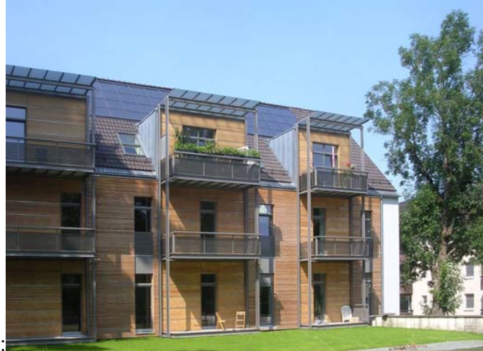
Figure 3: Net Zero Energy Buildings Cluster / retrofit projects. Renovated district in Bad Aibling (DE), design: Schankula-Architekten. New buildings generate an energy surplus to compensate negative balances of refurbished former military accommodation buildings from the 1930s. ST and PV areas differ significantly from each other. The shown example feed heat into the settlements local heating grid by means of 2000 m 2 of ST collectors. Source: Schankula-Architekten.
