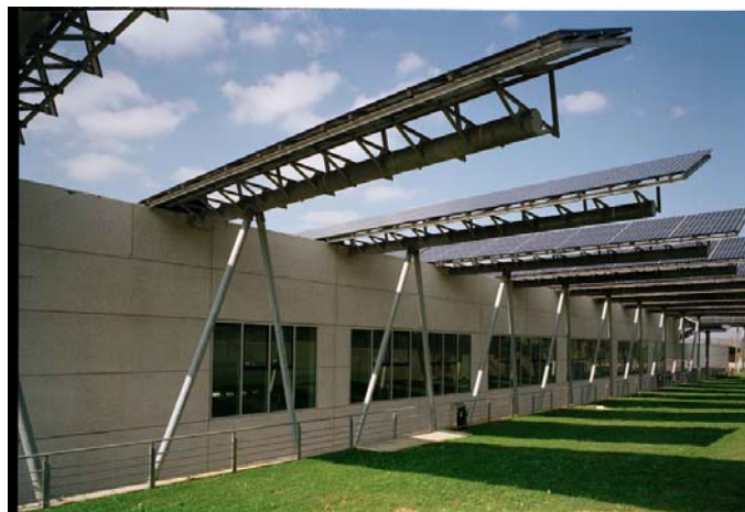
Figure 6: Efficient building by a compact structure or more solar usable surface area? Rainbow Headquarters, Loreto (IT), design: S. Bianchi & E. Straffi. PV modules are arranged as wings hanging over from the building’s physical boundary. Picture © L. Filateci.
